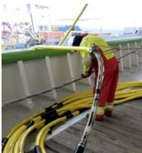
Installation of the DHSS during preparation of a new seismic vessel
