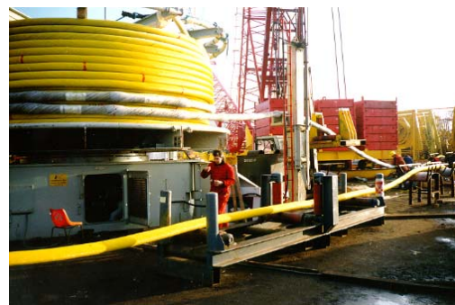
PMI Armor Rods applied on cable.
