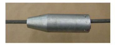
Slide the insert over the cable in the direction of the arrow as shown. Position this in the location where the DYNA-GRIP or EVERGRIP Termination is to be installed.
