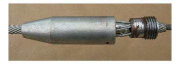
11. PMI recommends using thread lubricant or antiseize compound on the retainer and adaptor threads to aid in future disassembly.
